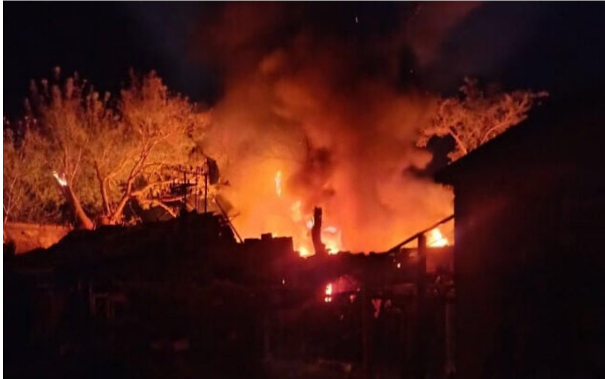
A Russian drone strike on the Nachlas Eliezer Synagogue in the Peresyp district of Odesa, Ukraine, on August 4, 2025, caused significant damage to the building. (Rabbi Pinchas Goldschmidt/X)
